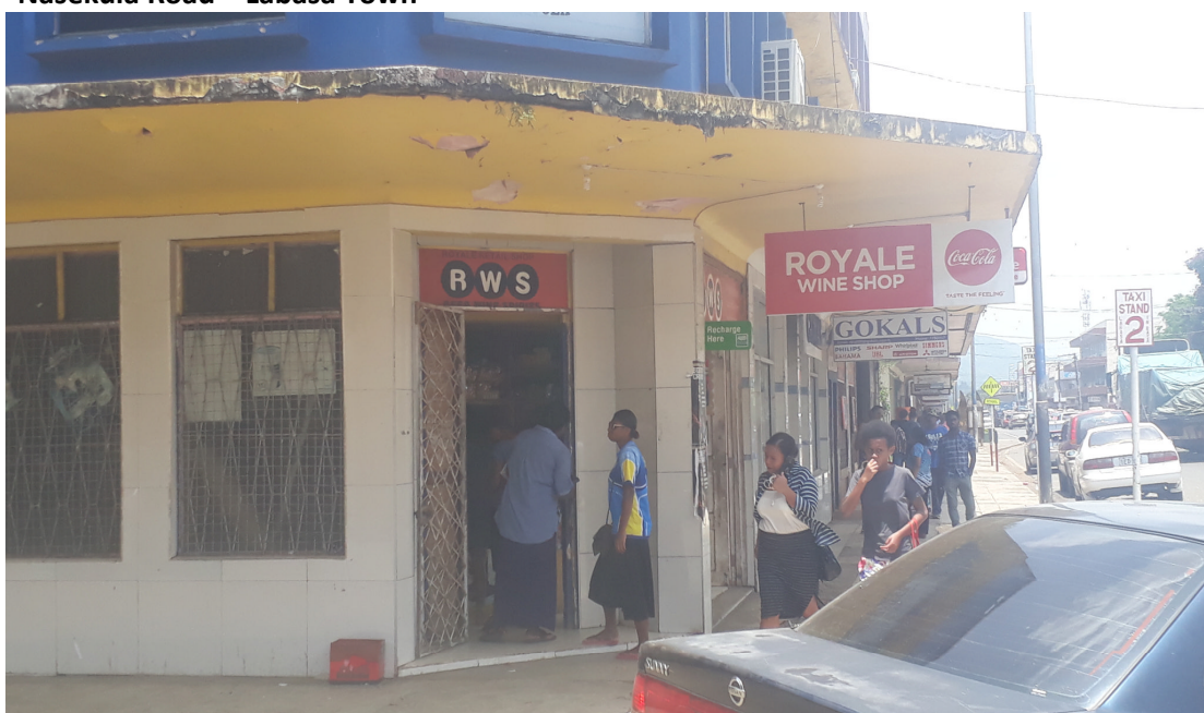
Photograph T1 - Taken by Departmental Officers at 1.15pm 1 December 2018 Nasekula Road – Labasa Town 9
